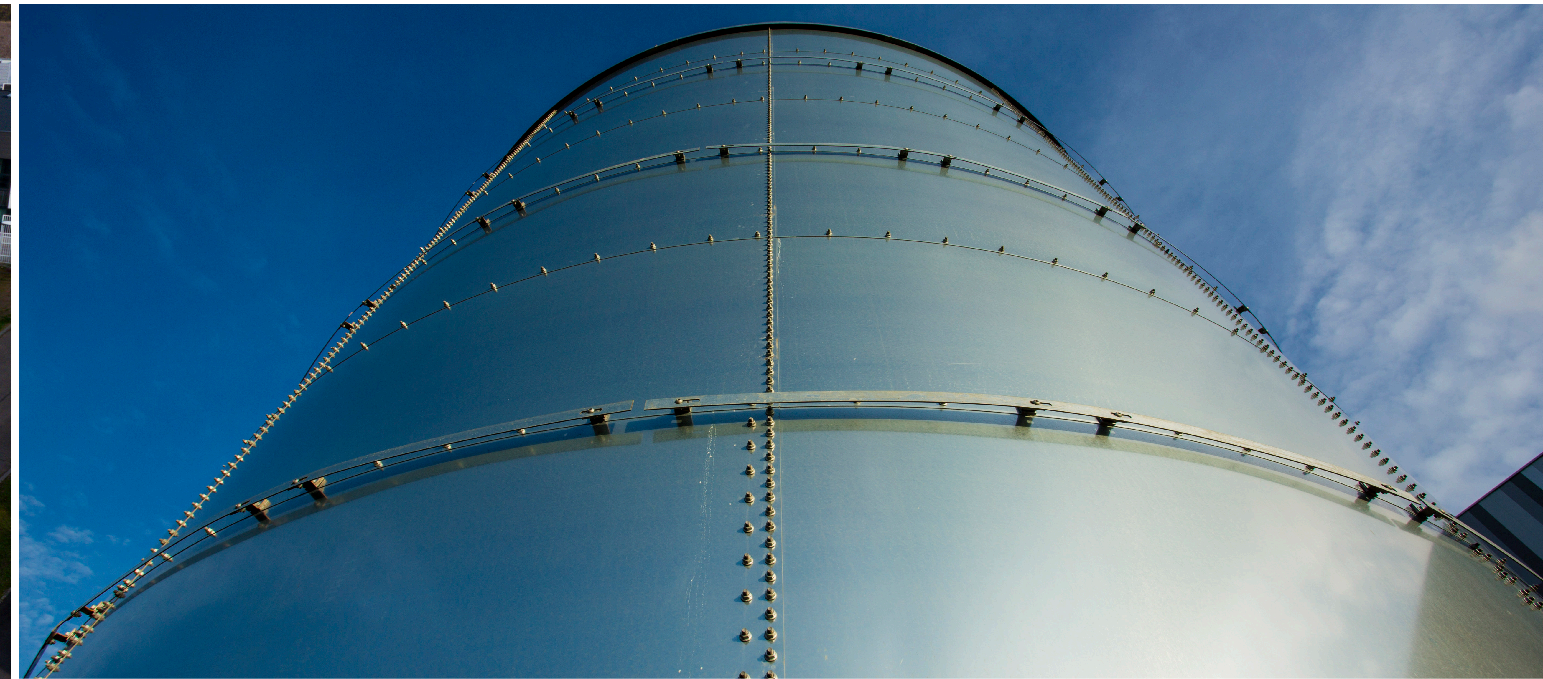
Water tank/Cuve 550 m 3
